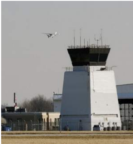
Tower at Bowman Field. Feb. 23, 2013
